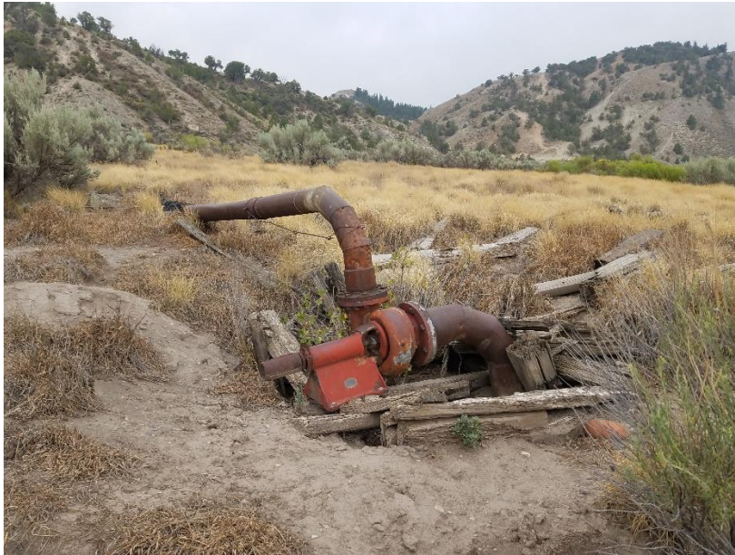
Photo 10. Abandoned pipeline parts.
