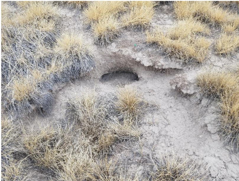
Photo 2. Evidence of erodible silty soils.
