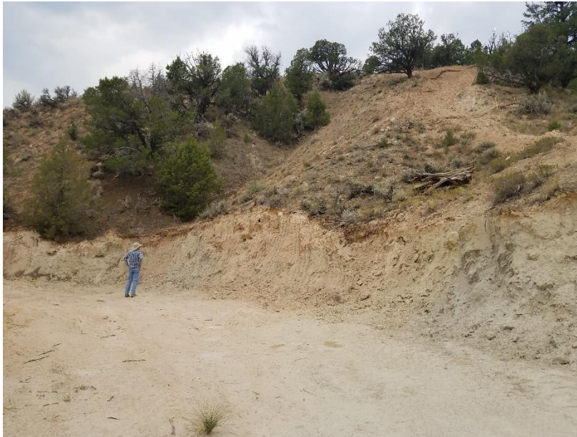
Photo 3. Highly weathered Eagle Valley Evaporite exposure along service road leading to Hockett Gulch.
