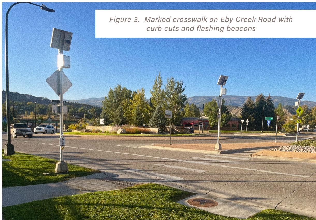
*Figure 3. Marked crosswalk on Eby Creek Road with curb cuts and flashing beacons*
