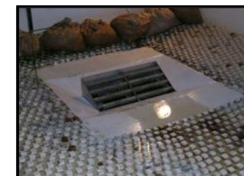
CDOT Type D Inlet Parallel (30" Inlet & Depressed)
